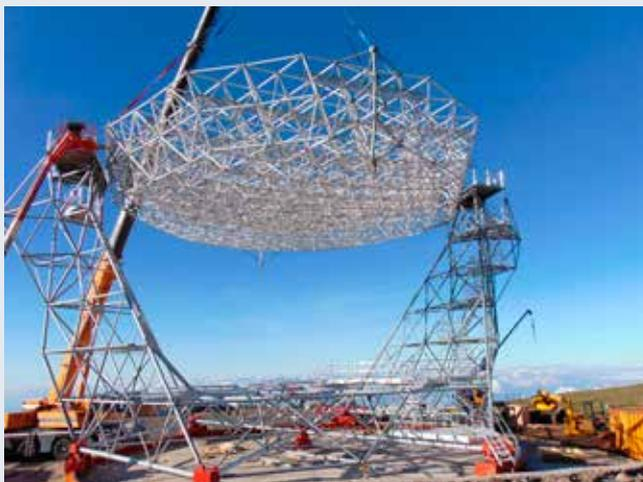
Installation of mechanical support for the mirror of the first large telescope of the CTA observatory at La Palma, Spain, in December 2017.
